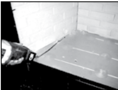
Figure 12.2 - Using a saws-all, cut out the floor.
