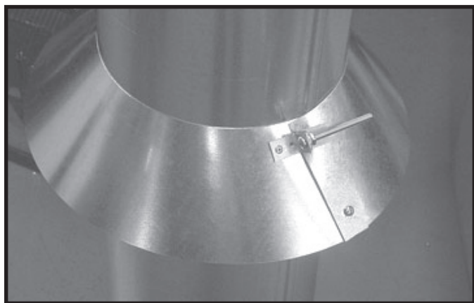
Figure 7.13 insert Bolt into Brackets
