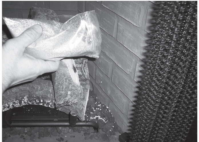
Figure 14.22 Placement of Vermiculite
