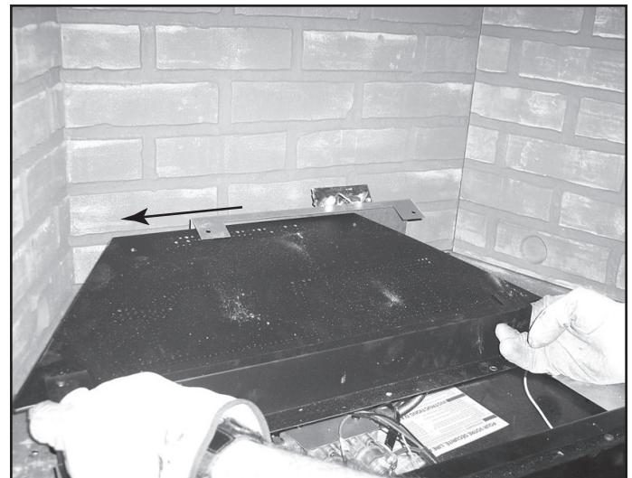
Figure 14.30 Side Burner Assembly to Left
