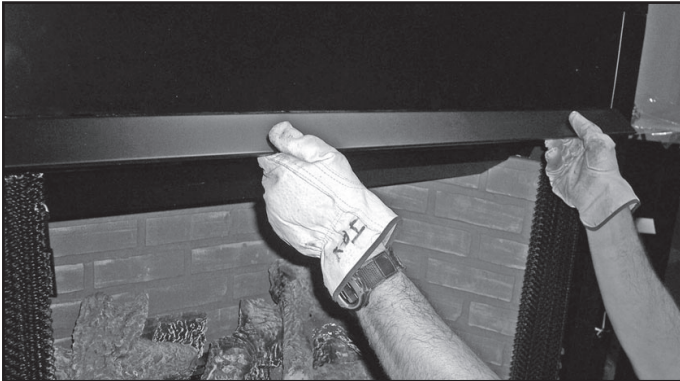
Figure 14.27 Installing the Hood
