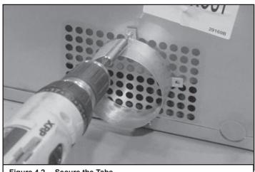
Figure 4.2 Secure the Tabs
