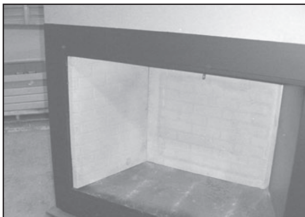
Figure 8.6 Side Refractory Installed
