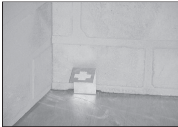
Figure 8.8 Grate Retaining Bracket in Place
