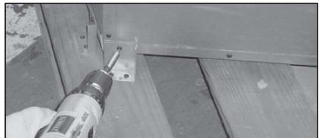
Figure 3.11 Removing Shipping Brackets
