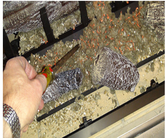
Figure 9- Adjusting of Flame Pattern
