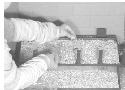
Figure 7 Placing Rock Wool
