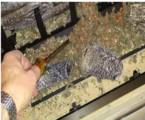
Figure 6- Adjusting of Flame Pattern
