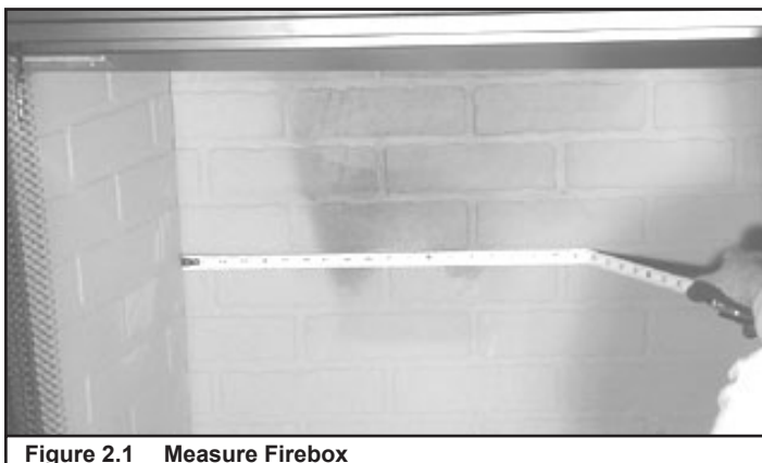
Figure 2.1 Measure Firebox
