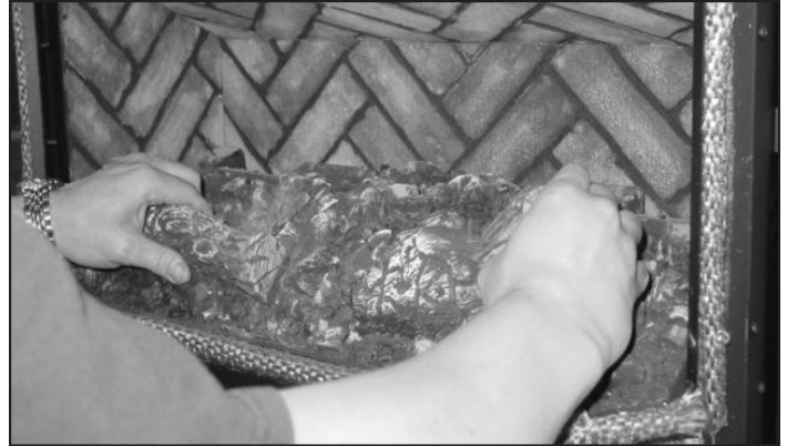
Figure 6.2 - Lift burner up and out of the firebox opening.
