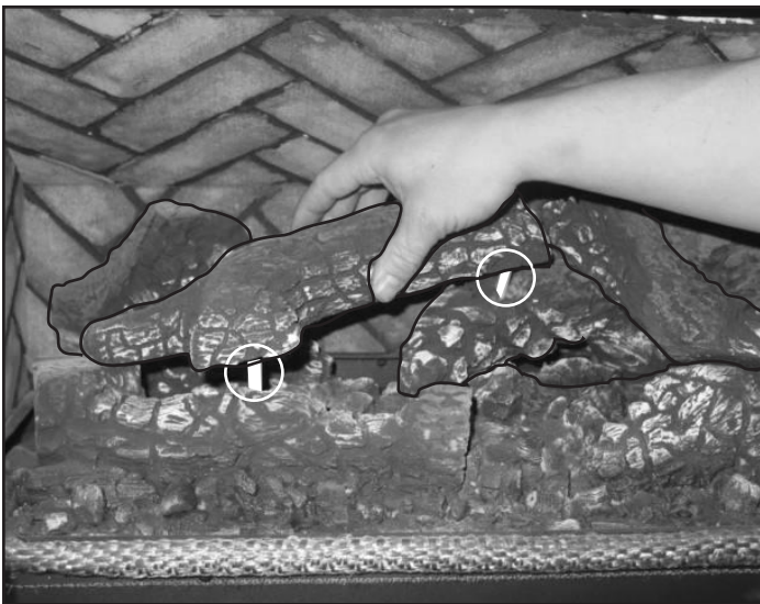
Figure 8.23 - Install the left twig (#6) over the locator pins in the right rear log and the left front log.
