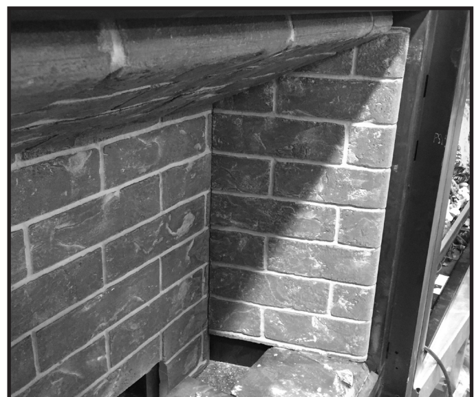
Figure 11.6 Right Refractory Panel Installed
