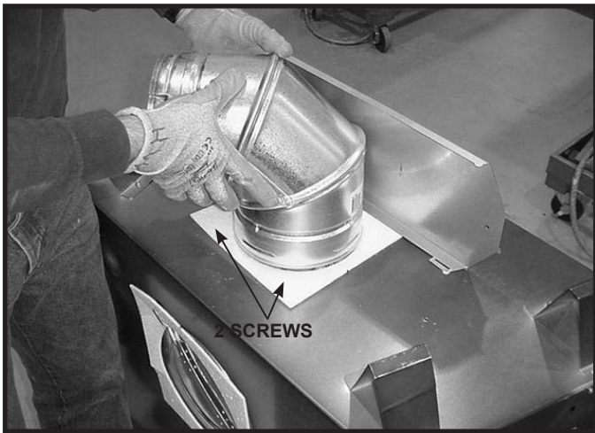
Figure 6.7 To attach the first section of vent pipe, make sure to use the fiberglass gasket to seal between the first vent component and the outer fireplace wrap. Use 2 self tapping screws to secure the gasket to the outer wrap.
