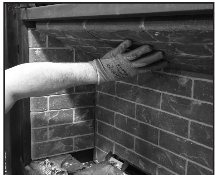
Figure 11.5 Install Right Refractory Panel
