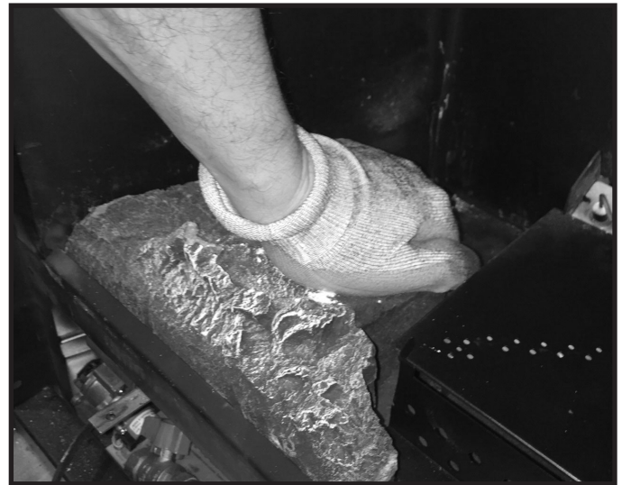
Figure 11.1 Press Left Hearth Firmly Into Place
