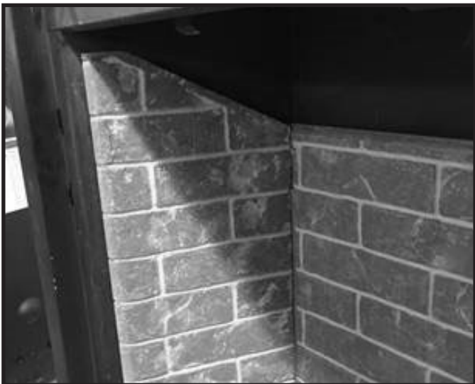
Figure 11.3 Install Left Refractory Panel
