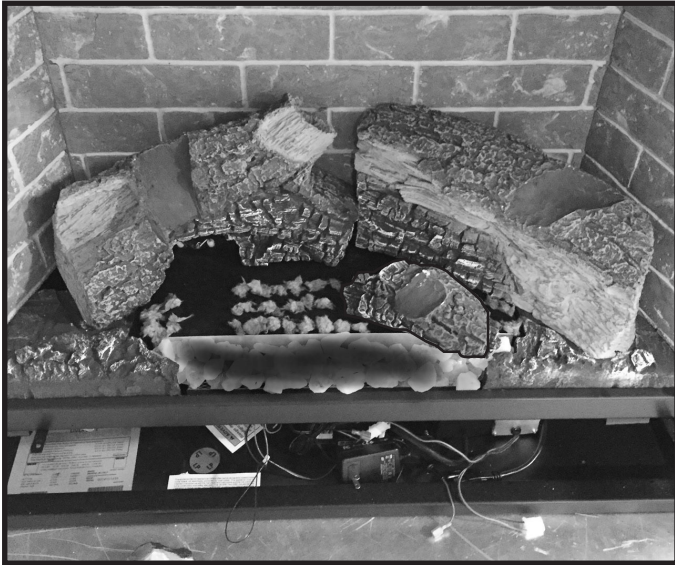
Figure 6. Burner Log Installed
