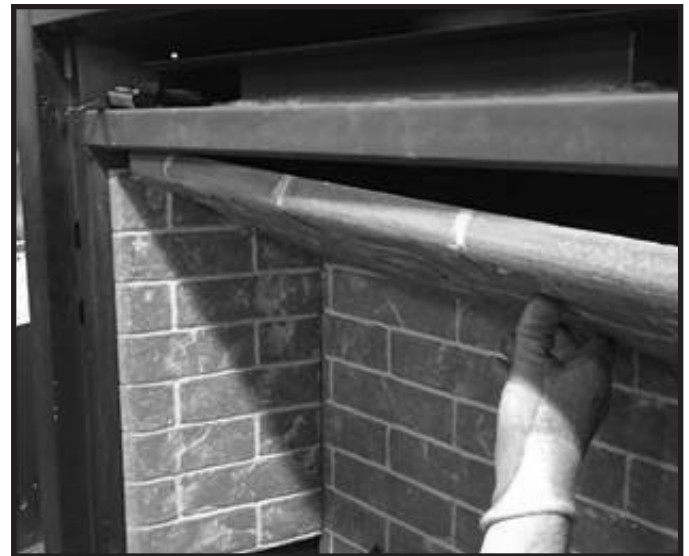
Figure 11.4 Install Top Refractory Panel
