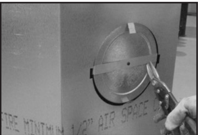
Figure 6.9 (Generic Fireplace Shown) Cut the metal retaining band and fold the sides out.
