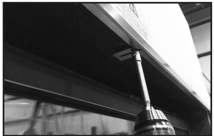
Figure 10.5 Install Trim Ring
