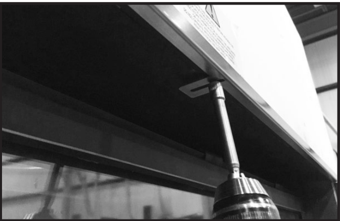
Figure 10.5 Install Trim Ring
