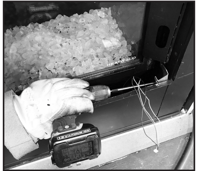
Figure 5.2 Remove Existing Glass Mounting Brackets (If Installed)
