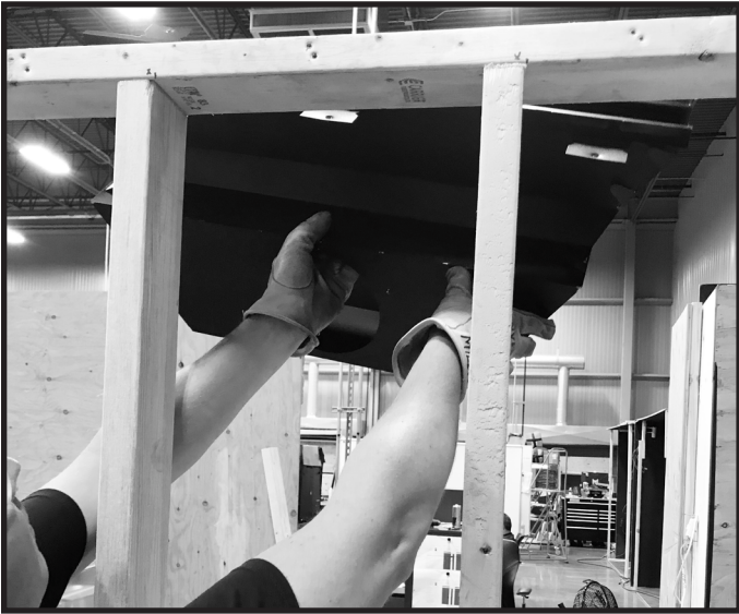
Figure 6.7 Rotate Plenum to Horizontal Orientation
