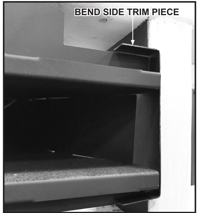
Figure 6.15 Bend Side Trim Piece
