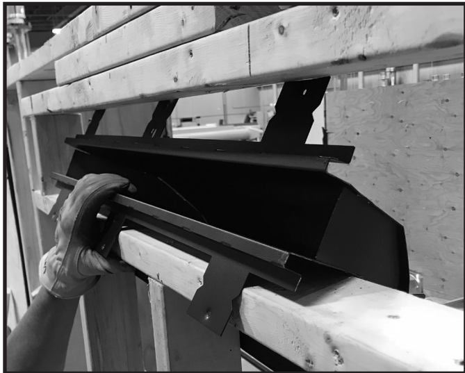
Figure 6.8 Place Plenum From Inside of the Chase
