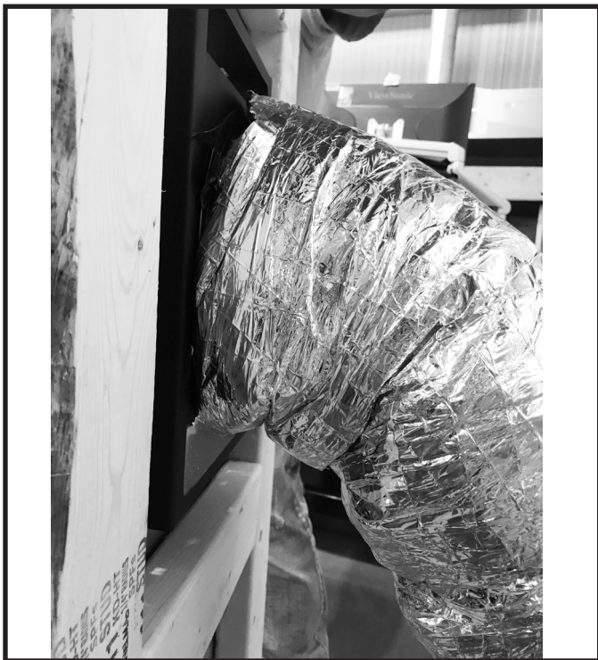
Figure 7.6 Install Flex Venting to Side Discharge Assembly
