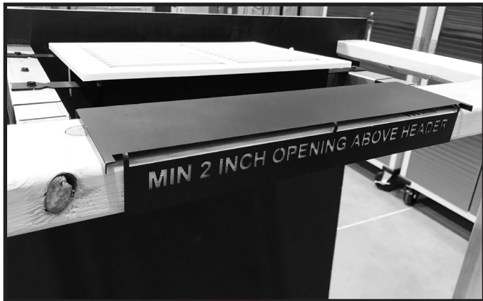
Figure 8.21 Heat Shield Centered and Mounted
