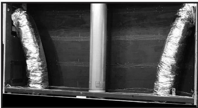
Figure 7.7 Flex Venting Installed
