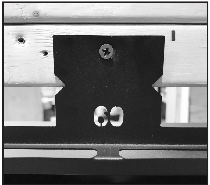
Figure 6.10 Secure Nailing Tabs
