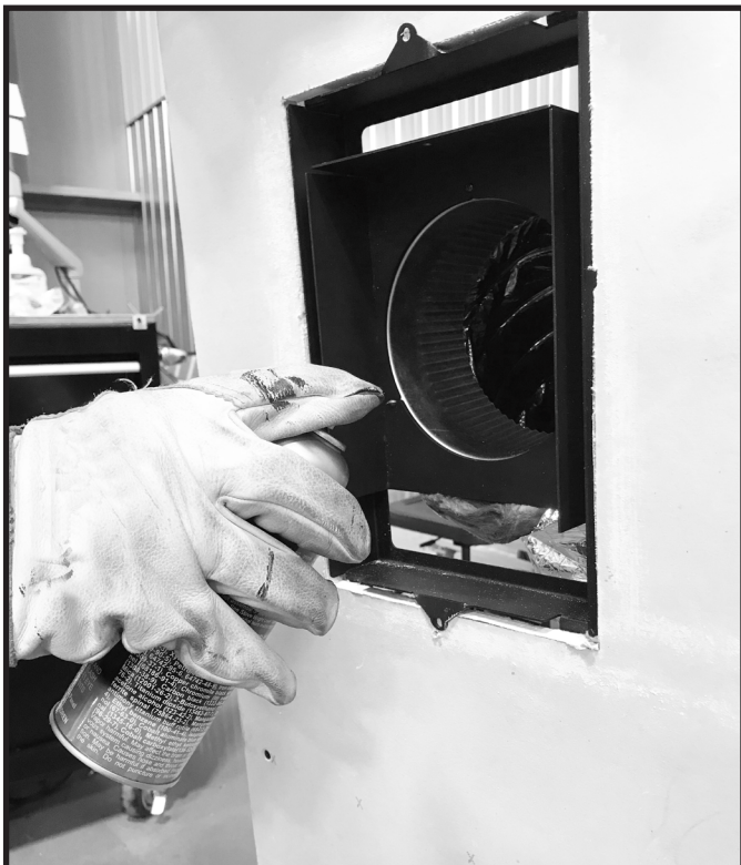
Figure 7.11 Paint Outer Wrapping of Flex Vent (Optional)
