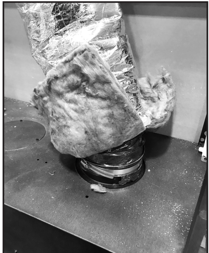
Figure 8.24 Install Flex Venting to Appliance
