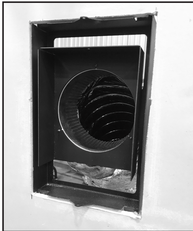
Figure 7.8 Wall Sheathing Installed
