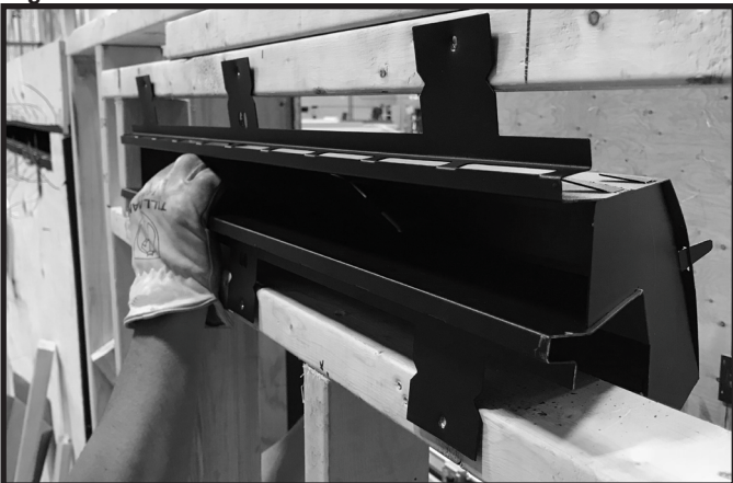
Figure 6.9 Position Plenum
