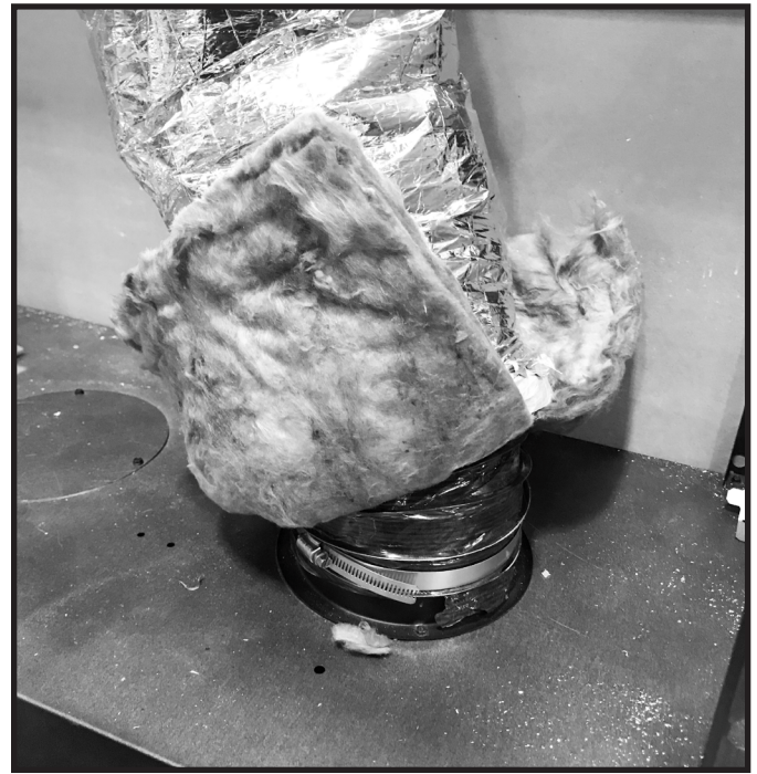
Figure 7.4 Install Flex Venting to Appliance
