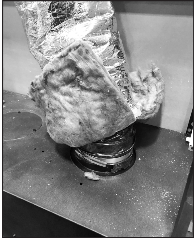
Figure 6.18 Install Flex Venting to Appliance
