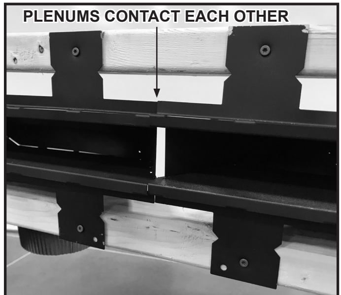
Figure 6.12 Plenums Contact Each Other
