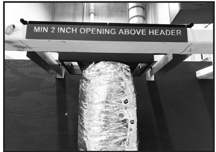
Figure 8.23 Install Flex Venting to Appliance
