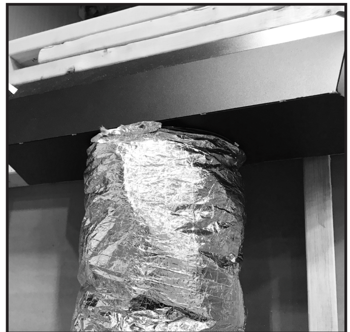
Figure 6.17 Install Flex Venting to Collar on Bottom of Plenums
