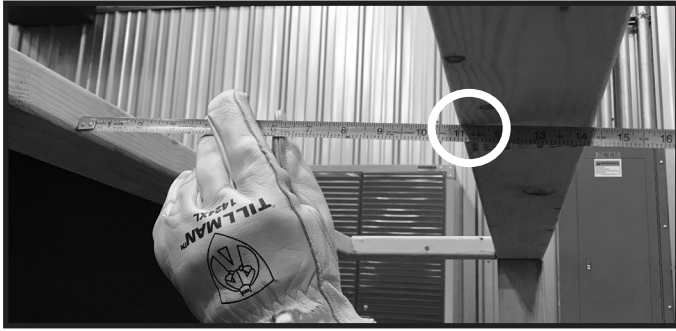
Figure 8.3 Measure Chase Depth
