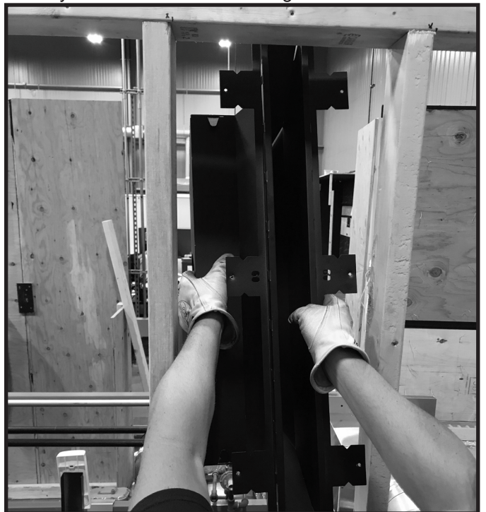
Figure 6.6 Turn Plenum Vertically to Clear Framing Studs
