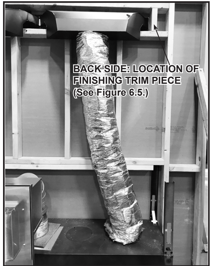
Figure 6.20 Flex Vent Installed with No Kinks
