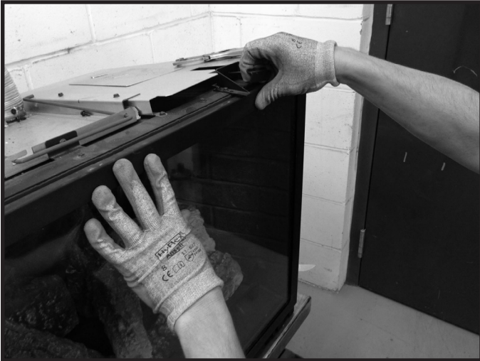
Figure 4.3 Release Glass Latches One at a Time
