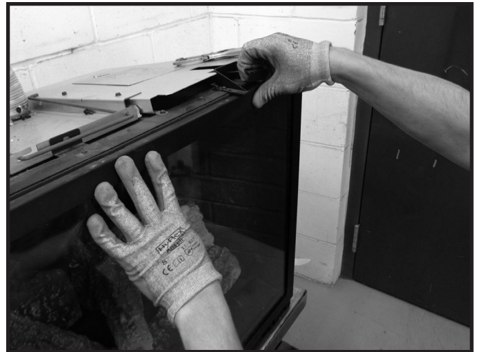
Figure 11.3 Release Glass Latches One at a Time
