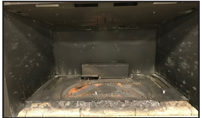
Figure 3 Base Refractory Installed
