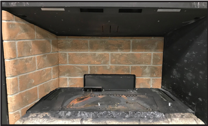
Figure 5 Left Refractory Installed
