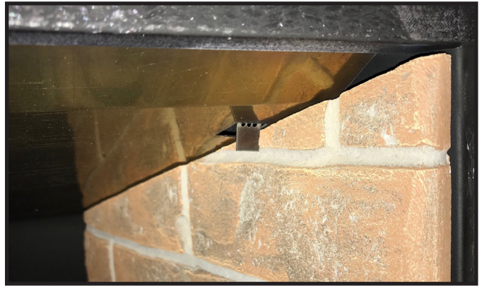
Figure 7 Right Refractory Handbend Tab
