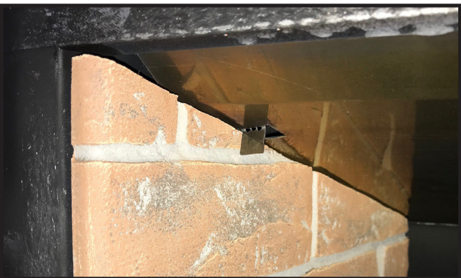
Figure 6 Left Refractory Handbend Tab
