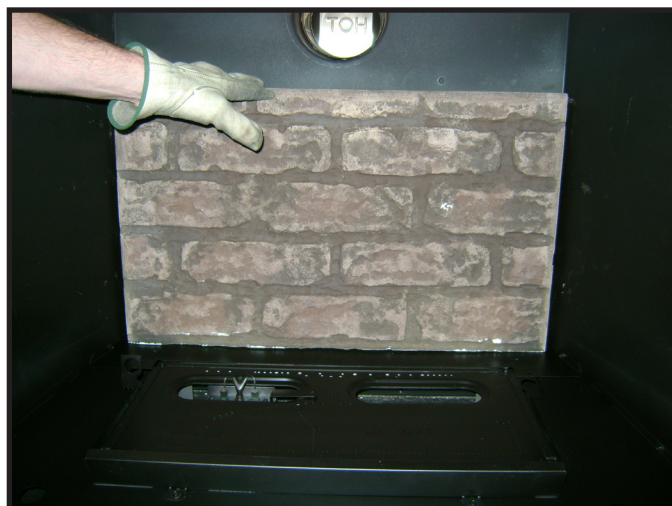
Figure 4.5 Back Refractory Removal
