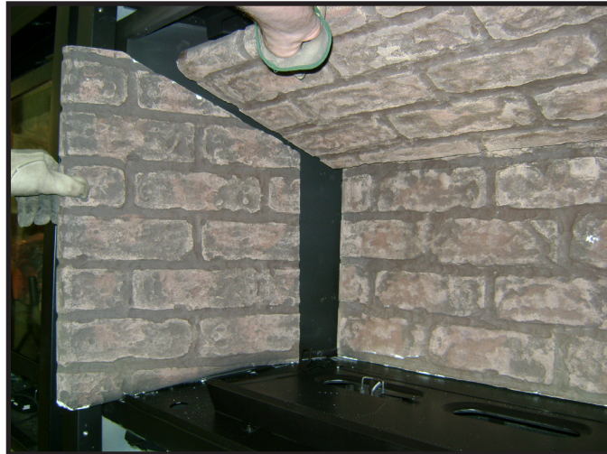
Figure 4.3 Top Refractory Removal
