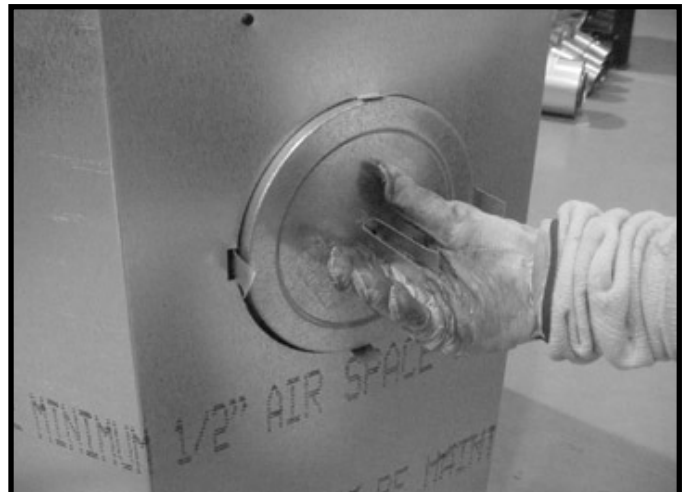
Figure 6.9 (Generic Fireplace Shown) Fold the center parts of the retaining band out and use to remove the seal cap.
