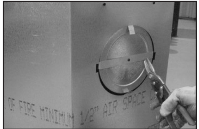
Figure 6.8 (Generic Fireplace Shown) Cut the metal retaining band and fold the sides out.
