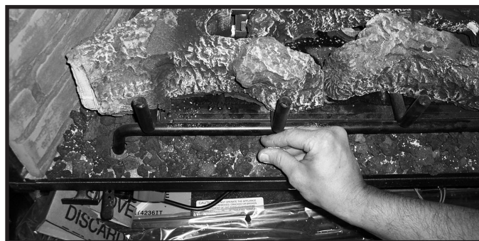
Figure 11.5 Placement of Vermiculite
