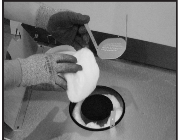
Figure 6.4 (Generic Fireplace Shown) Remove the insulation basket and white insulation from the center vent
