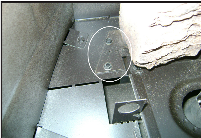
Figure 4.5 Remove Screws from Log Tabs
