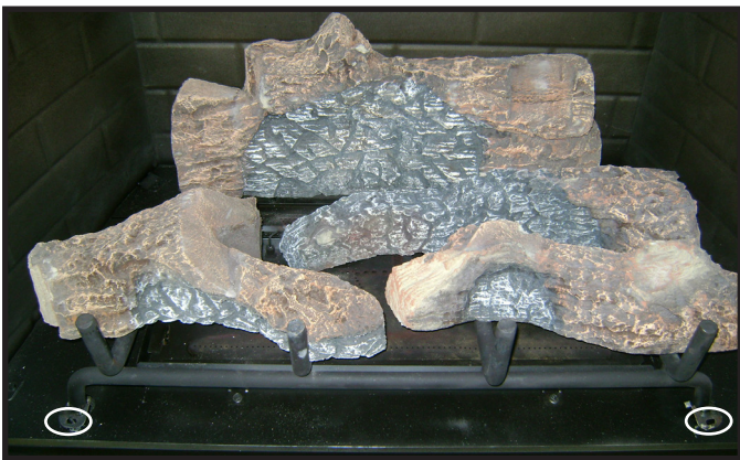
Figure 4.4 Remove Screws from Front Tab
