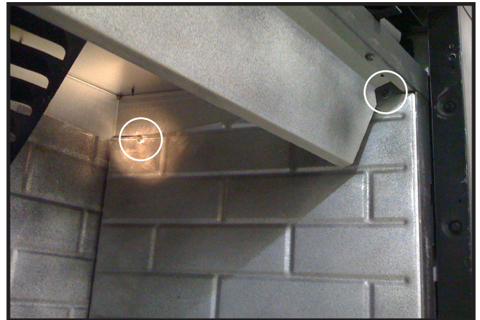
Figure 4.7 Top Screws For Metal Refractory
