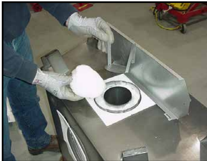
Figure 6.6 Remove the insulation basket and white insulation from the center vent pipe.
