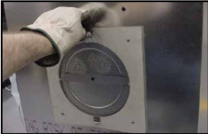
Figure 6.8 Fold the tabs toward the center of the fire plug (90°) and remove the insulation gasket.
