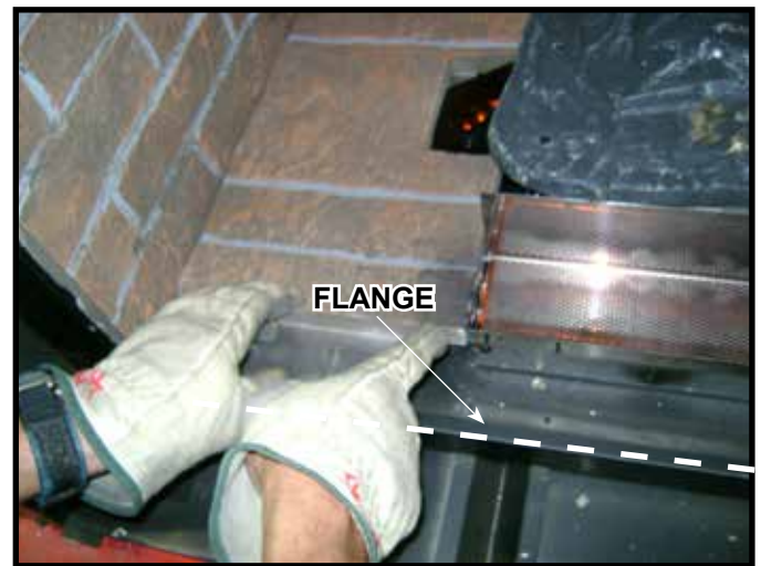
Figure 11.18 Positioning Left and Right Middle Base Refractory
