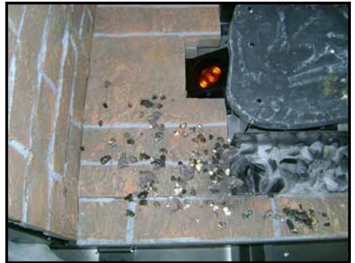
Figure 11.23 Ember Placement on Base Refractory
