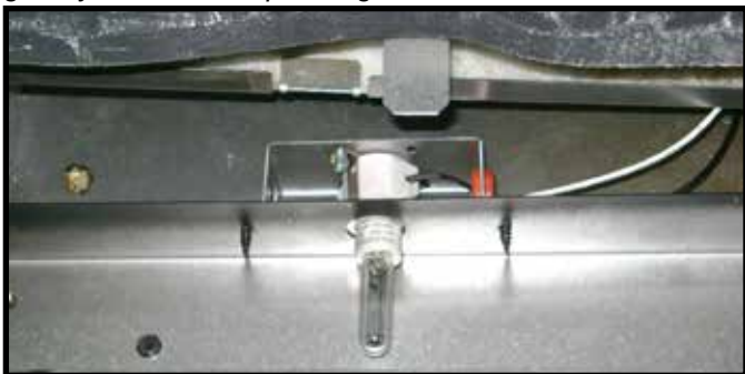
Figure 11.10 Ember Light Bulb Installed
