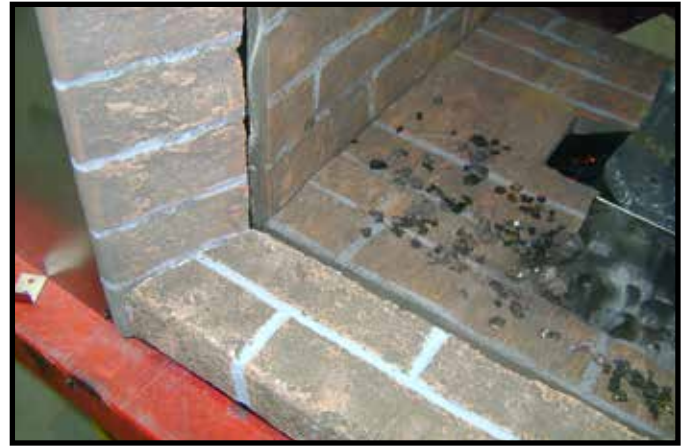
Figure 11.29 Outer Hearth Installation
