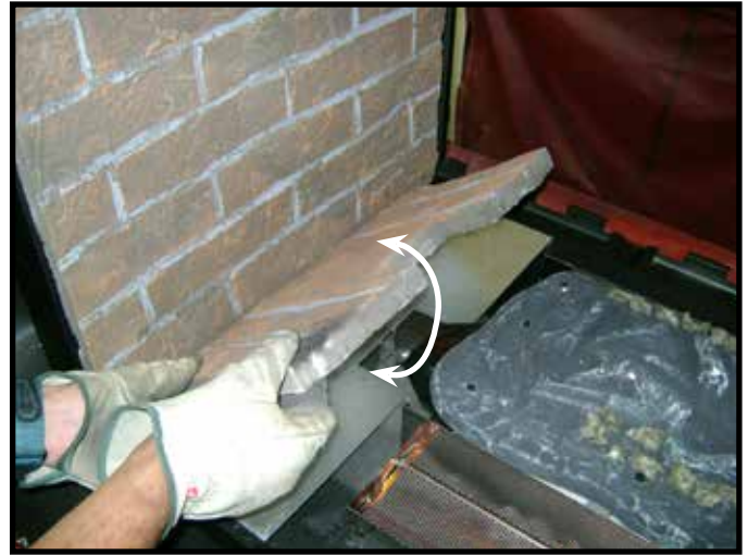
Figure 11.17 Positioning Inner Bottom Refractory
