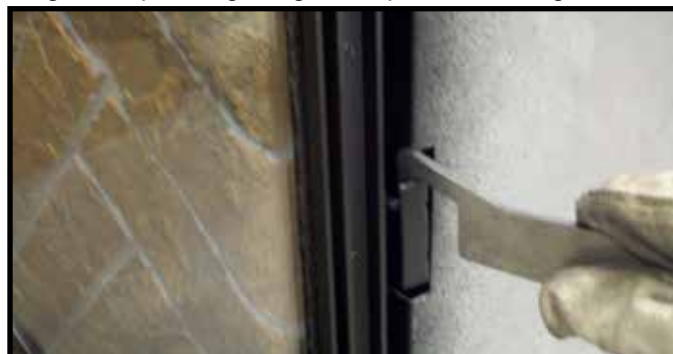
Figure 11.7. Securing Side Glass Clips
