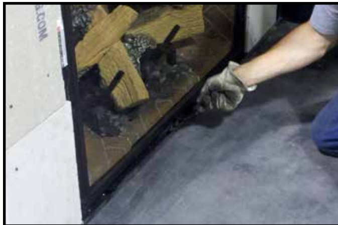
Figure 11.8. Securing Bottom Glass Clips
