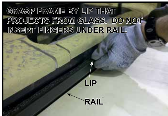
Figure 11.6. Installing Glass
