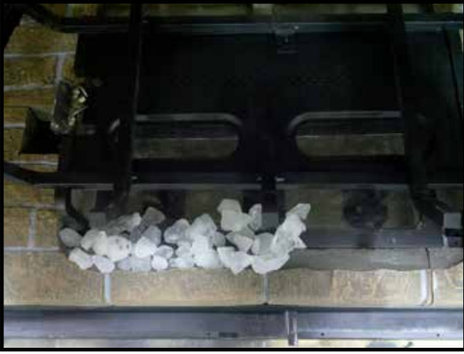
Figure 11.19. Install Teco-Sil
