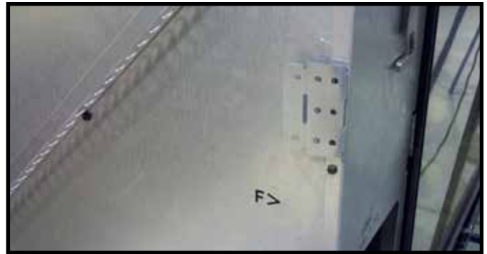
Figure 6.4 Side Nailing Tab in Shipping Position
