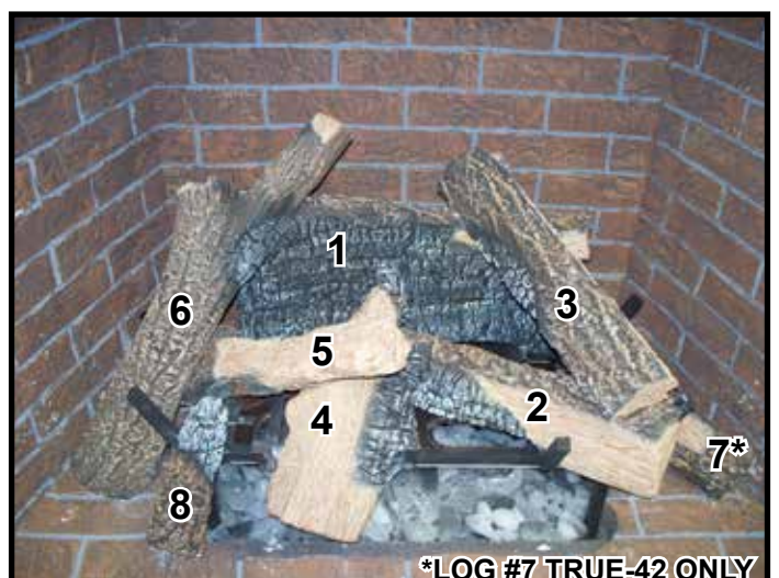
Figure 16. Log Set Installed.
