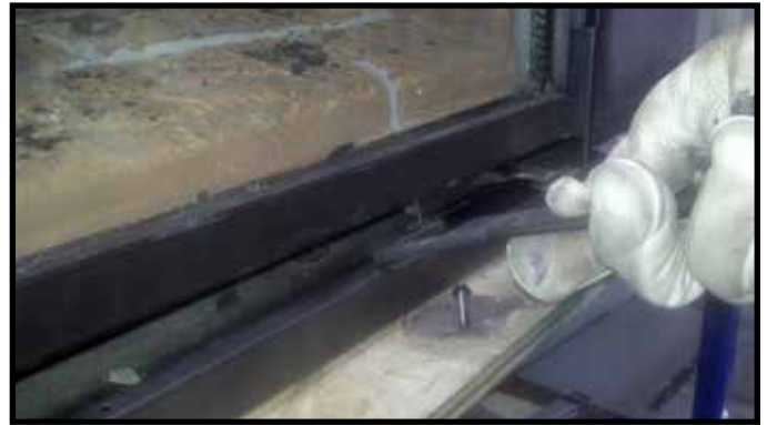
Figure 11.2. Glass Clip Tool Location
