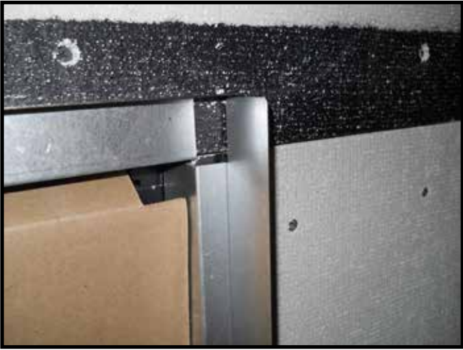
Figure 10.5 Finishing Template Bends
