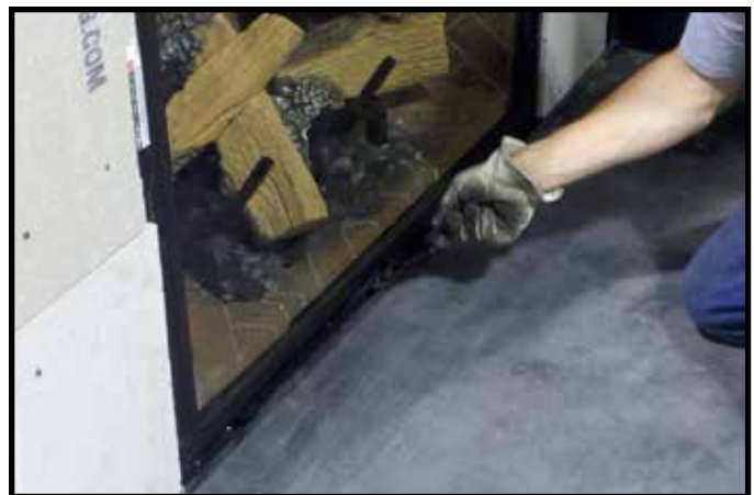
Figure 11.8. Securing Bottom Glass Clips
