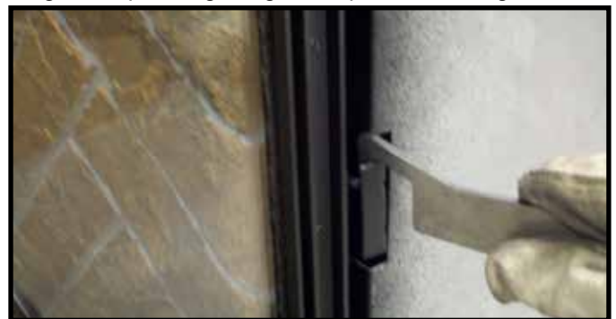
Figure 11.7. Securing Side Glass Clips
