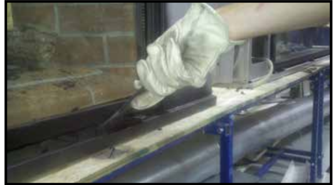
Figure 11.3. Inserting Glass Clip Tool
