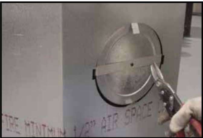
Figure 6.10 (Generic Fireplace Shown) Cut the metal retaining band and fold the sides out.
