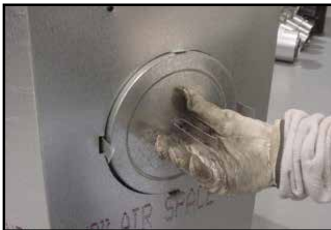
Figure 6.11 (Generic Fireplace Shown) Fold the center parts of the retaining band out and use to remove the seal cap.
