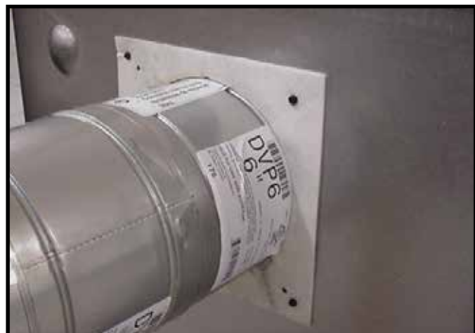
Figure 6.13 (Generic Fireplace Shown) Attach the first vent section (it will snap into place). Slide the insulation gasket onto the vent section, up against the appliance and over the tabs. Use two self-tapping screws to secure gasket to outer wrap.
