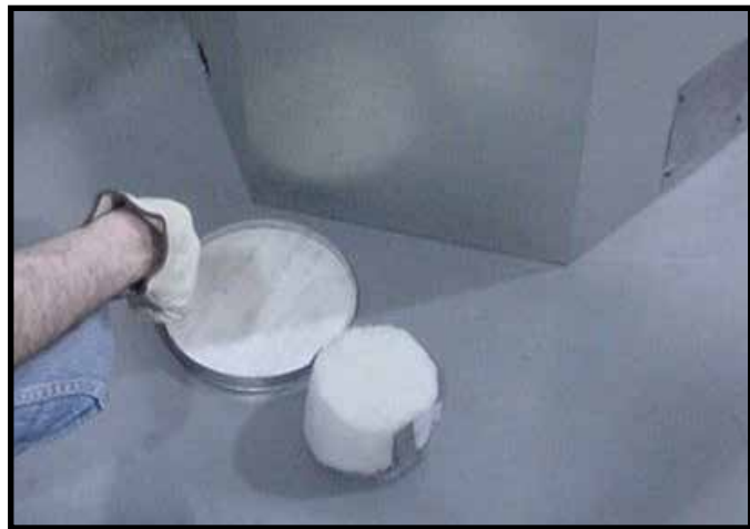
Figure 6.12 (Generic Fireplace Shown) Discard the seal cap, remove and discard the insulation basket. Note: Once the seal cap has been removed it CANNOT be reattached.
