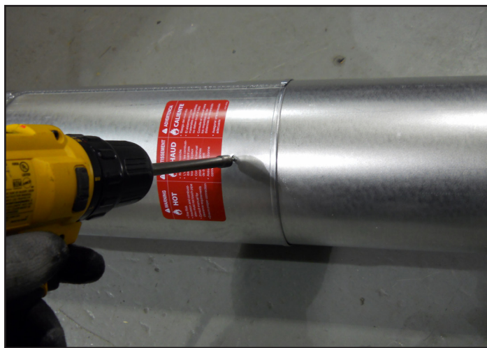
Figure 7.4 Vis de la section coulissante
