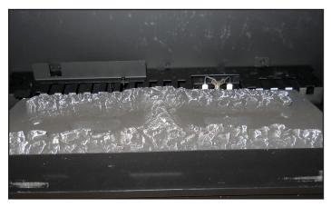
Figure 10.6 - Install Rear Refactory
