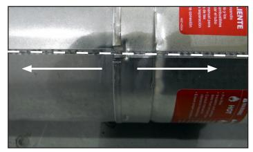
Figure 7.8 - Align and Disassemble Vent Sections
