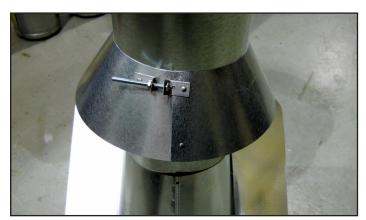
Figure 7.14 - Insert Bolt into Brackets
