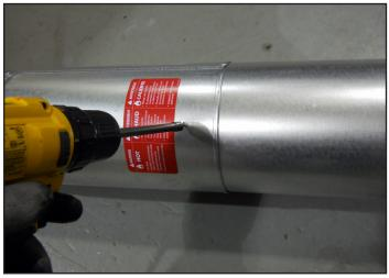
Figure 7.4 - Screws into Slip Section
