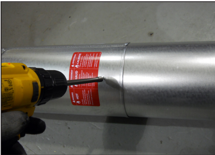
Figure 7.4 - Screws into Slip Section
