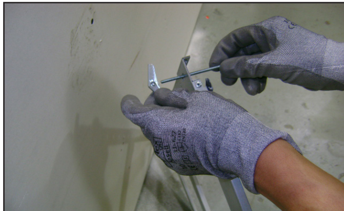
Figure 4.10 Toggle Bolt Installation through Mounting Bracket
