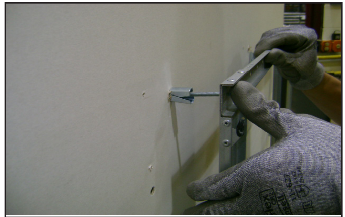
Figure 4.6 Installing Anchors in Hollow Wall
