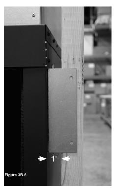
The nailing flanges will ensure the 1" minimum clearance is kept to combustible framing.
