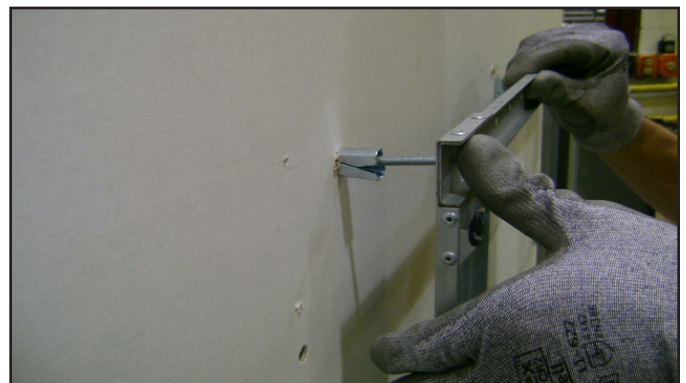
Figure 3 Installing Anchors in Hollow Wall
