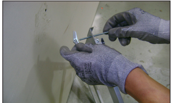
Figure 2 Toggle Bolt Installation through Mounting Bracket
